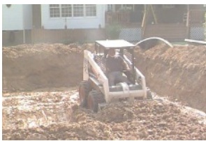
Digging with a bobcat
