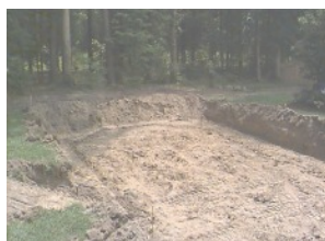
A finished initial dig on a rectangular pool.
