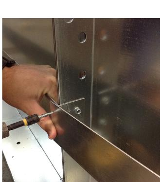
• 3. Pull the free end of the first support out and Repeat steps 1 and 2 at the next panel joint with a second skirting support.
